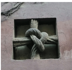
Fig. 2: Details of a knot on a wall in Prague
