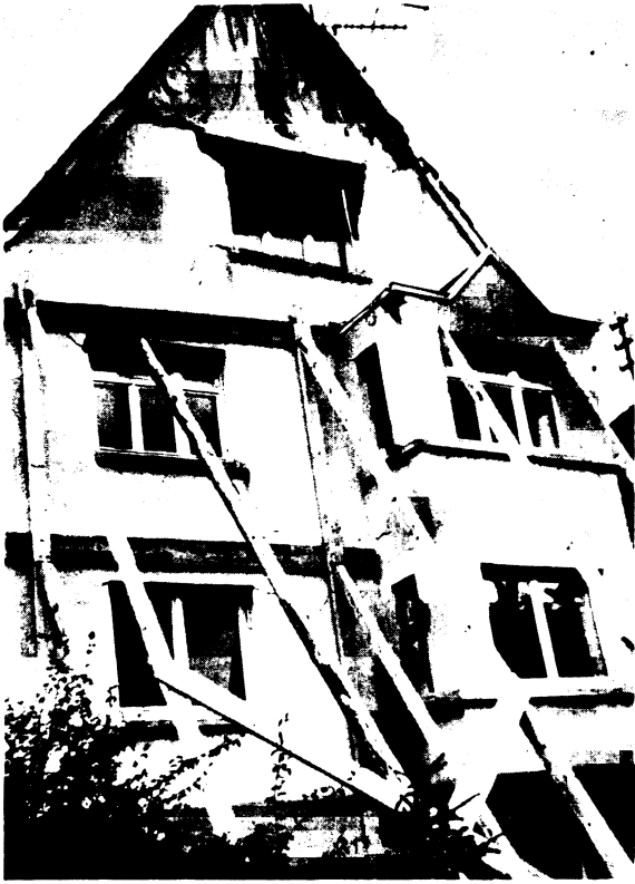
Fig. 1b The material damages caused by the earthquake of September 3, 1978 in Swabian Jura in Albstadt (FRG).
